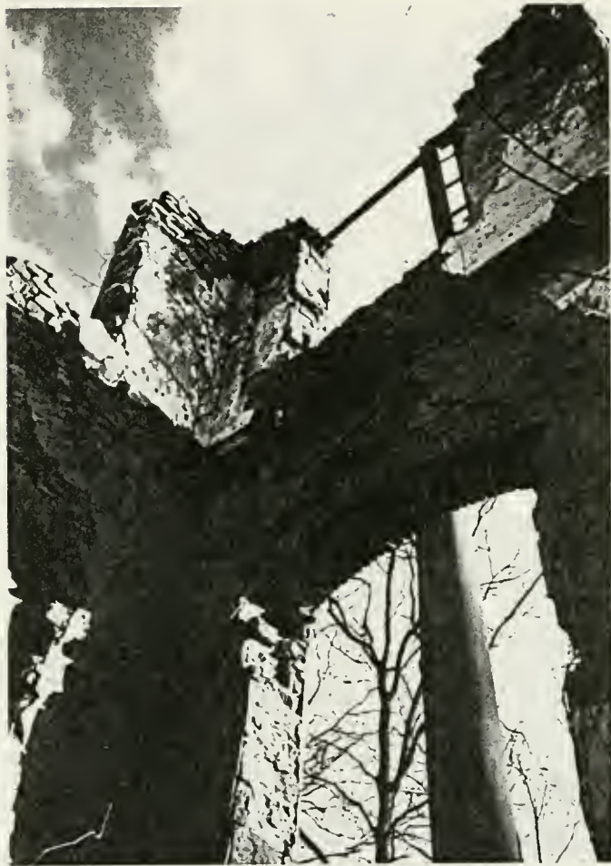
Figure 29: Interior view of archway shown in Figure 28
